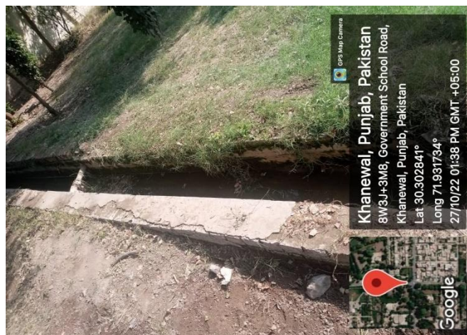
Figure 7: small water course at road 02
