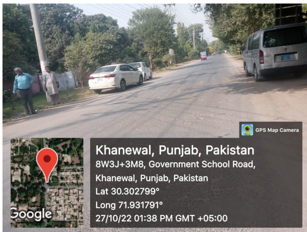
Figure 3: Road 02: condition of road
