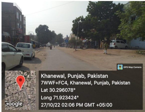
Figure 5: condition & RoW of Road 03
