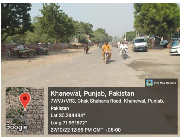
Figure 2: Road 01 condition of road and width RoW of Road
